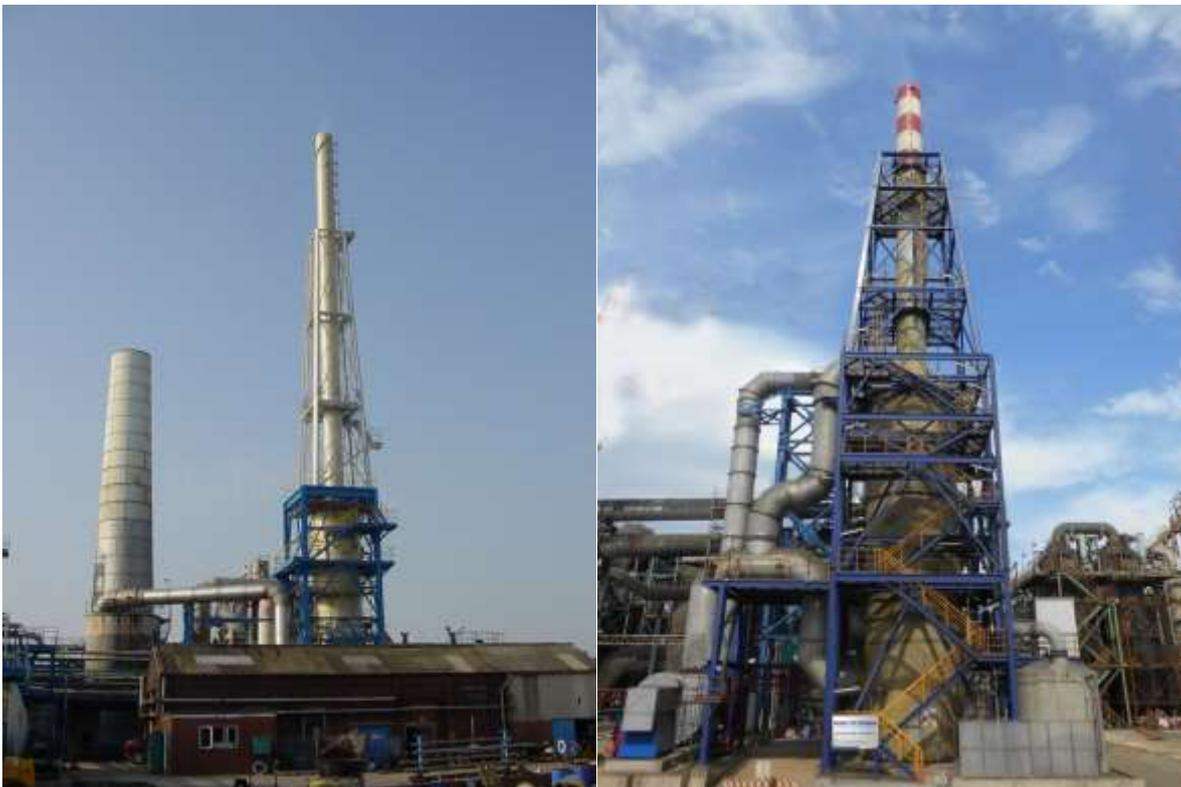
Pic. 18: SUPER<sup>OX</sup>-Processes downstream sulphuric acid plants
