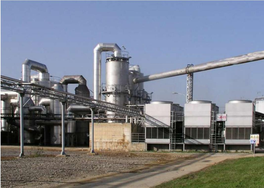
Pic. 9: Complete revamped Sulphuric Acid DC-Plant (600 tpd)
