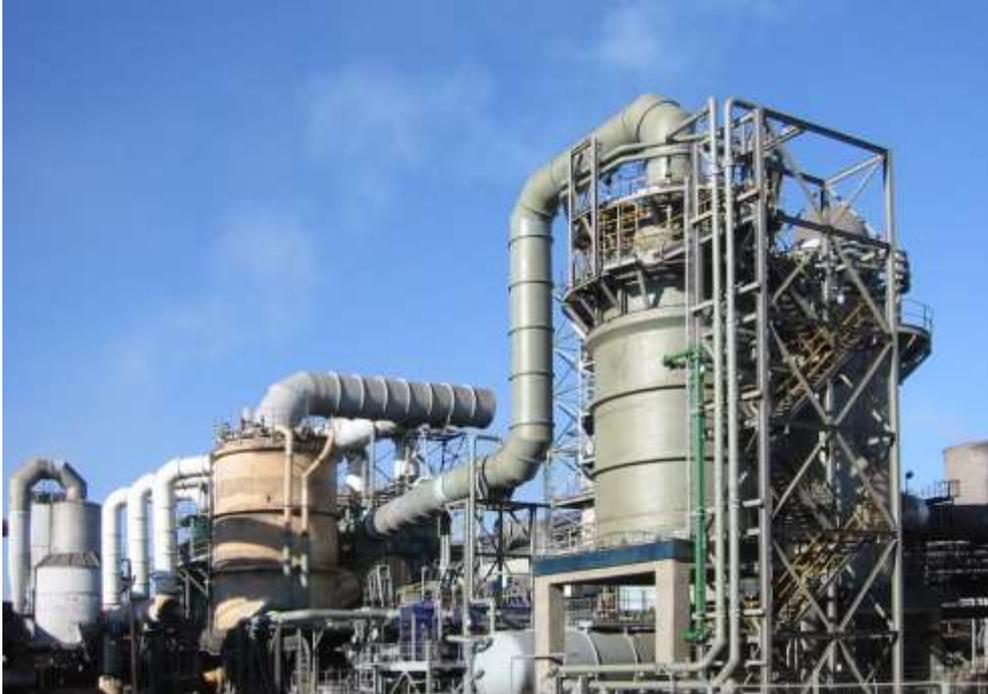
Pic. 4: Cleaning off gases by means of absorption and aerosol removal downstream of pyro-metallurgical processes in non-ferrous industries.
