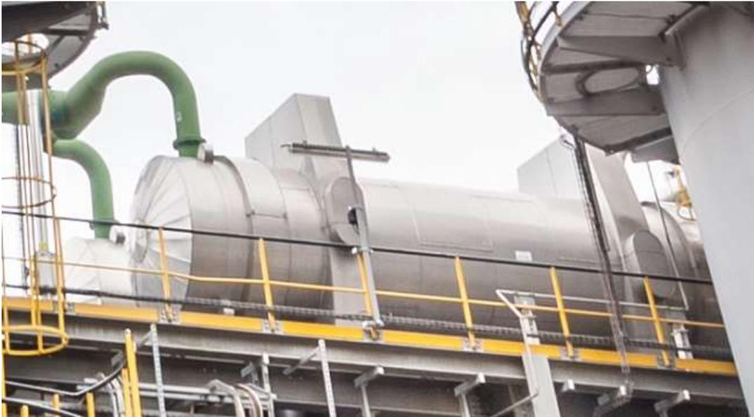
Pic. 16: Anodic-Protected-Acid-Coolers
