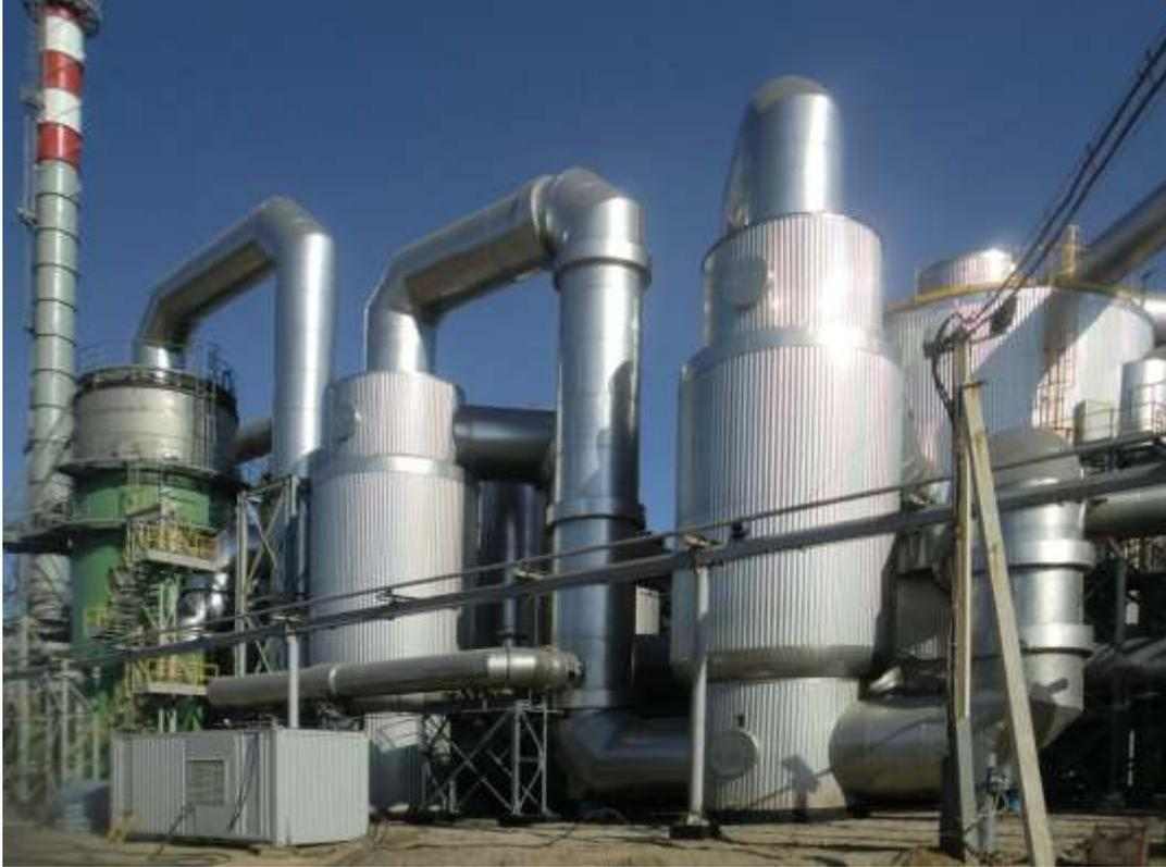
Pic. 7: 2,000 tpd Sulphuric Acid DC-Plant based on sulphur burning with THRC
