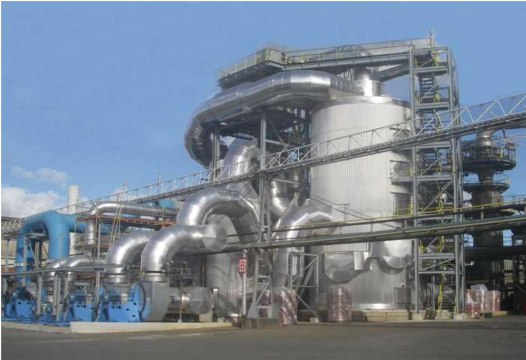
Pic. 13: Wet-Gas-Cleaning Plant down a Mo-roasting plant
